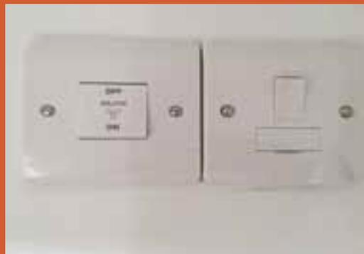
**Bathroom light switch for automatic boost of extract**
