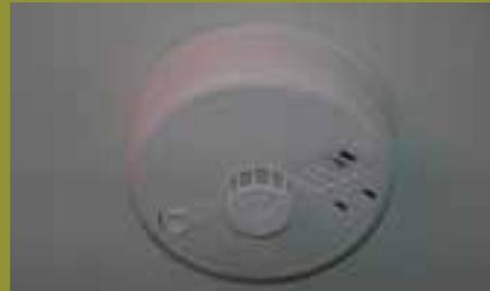
In addition to sounding in the event of a fire, your detector may give various audible indications of a malfunction. Please refer to the instruction leaflet in section 3 of this residents pack for details of how the detector functions and full clear instructions for the maintenance of this importance piece of equipment. **IT MAY SAVE YOUR LIFE.**
